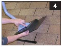
Install dish foot on deck plate with cap bolts
