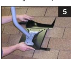
Lift upper shingle and slide deck plate under shingle, seat deck plate over base plate
