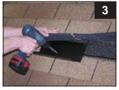
Install base plate with trusshead screws
