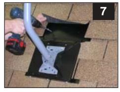
Lift shingle, install deck plate using trusshead screws, use small amount of roof cement under top shingle
