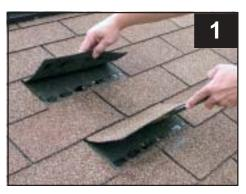
Locate truss with stud finder, lift shingles with prybar at dish location, do not lift middle row
