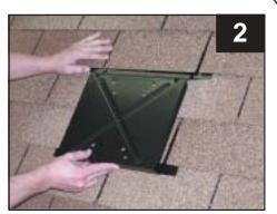
Before screwing base plate to roof, align both base & deck plate to assure shingles will fall into place
