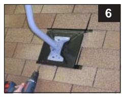
Use tek screws to secure deck plate to base plate
